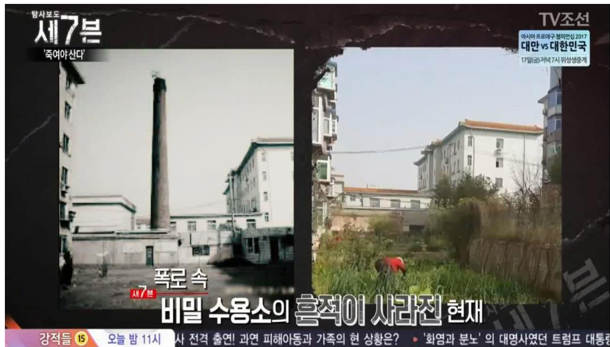
Left: boiler room and smokestack (photo taken over 10 years ago)
