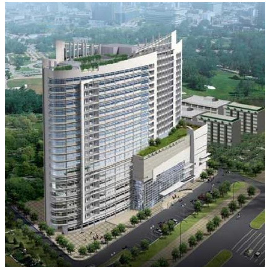
Third Xiangya Hospital's new surgery building with 1,000 beds
