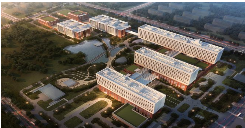
Rendering: Bird’s-eye view of the First Affiliated Hospital of Zhejiang University, Yuhang Branch 397
